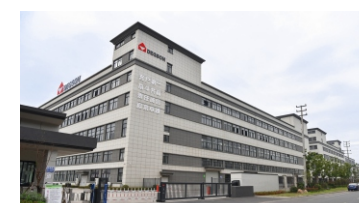
High-tech zone site
